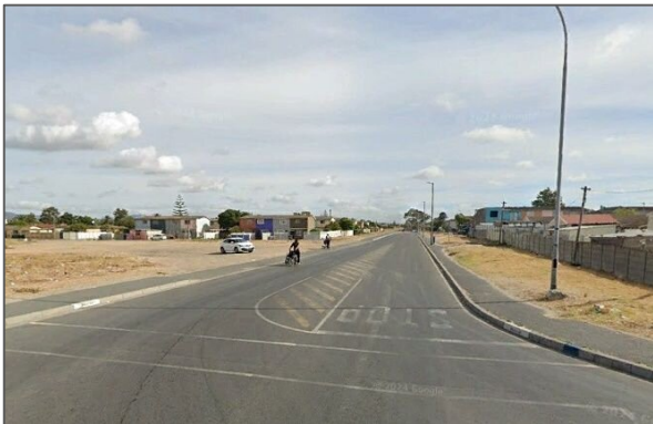
2a) Looking north along Reuter Street
