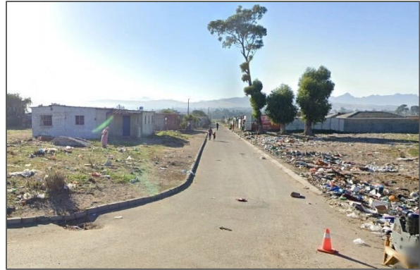
1b) Looking east along Verenigde Street
