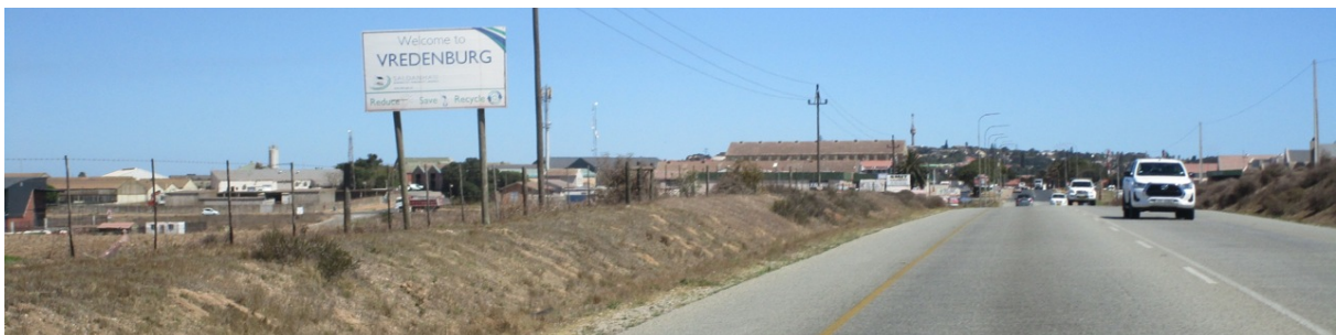
Photograph 4-33: R399 Southbound entering Vredenburg.
