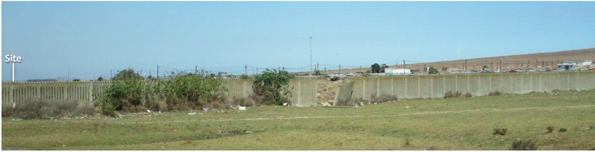
Photograph 4-15: R45 Eastbound from Vredenburg looking into the concrete fence.
