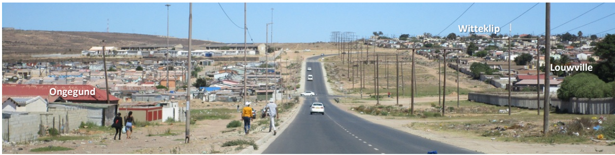
Photograph 4-24: Southern Bypass Southbound travelling between Ongegund and Louwville.
