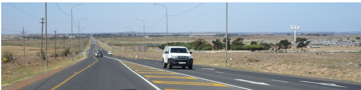
Photograph 4-14: R45 Eastbound from Vredenburg already passing the views to the site area.
