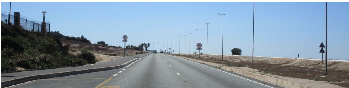
Photograph 4-34: R399 Northbound towards Vredenburg ex Weskus Mall.
