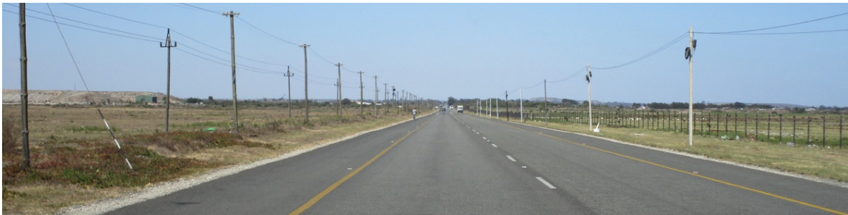
Photograph 4-21: R45 Eastbound from Vredenburg past the site towards the dump.
