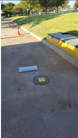
Photograph 3: Completed monitoring wells and headworks.
