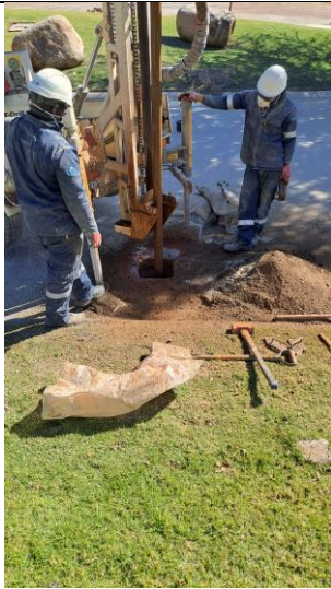
Photograph 1: Drilling in progress at the site.
