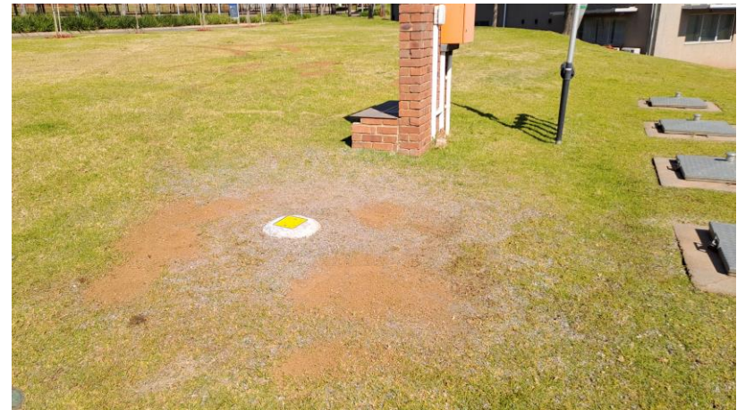
Photograph 4: Completed monitoring well and headworks.
