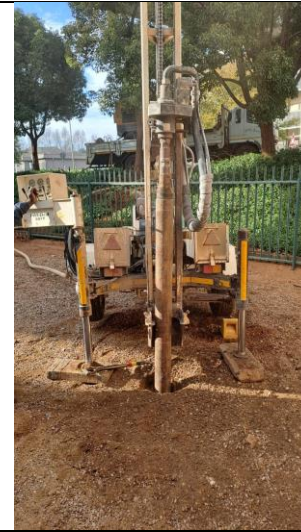
Photograph 2: General view of the drill rig during drilling.
