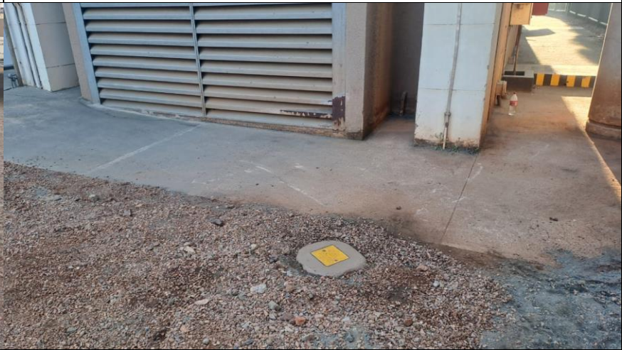
Photograph 4: Typical completed monitoring well and headworks.
