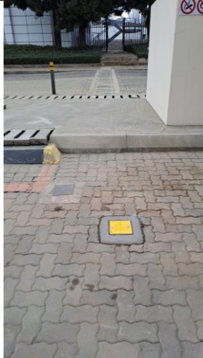
Photograph 3: Typical completed monitoring well and headworks.
