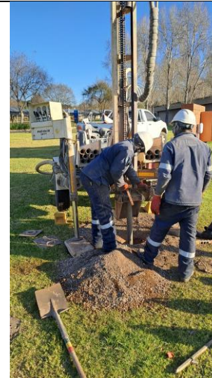
Photograph 2: General view of the drill rig during drilling.
