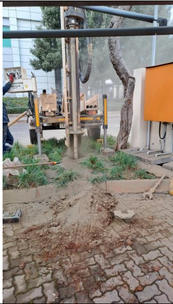
Photograph 1: General view of the drill rig during drilling operations.
