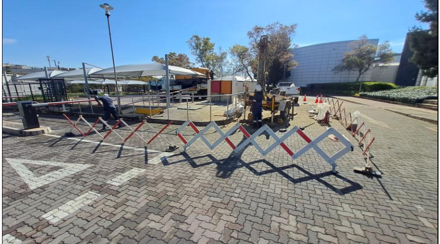
Photograph 2: General view of the Nexus tank farm during drilling operations.
